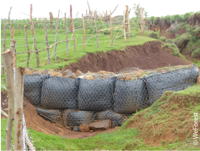
Building check dams to stop soil erosion.
